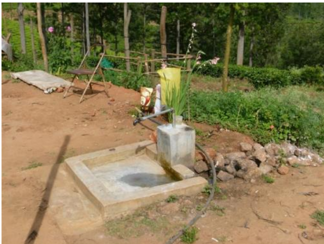
Upgrading of water pipes at certified estate
