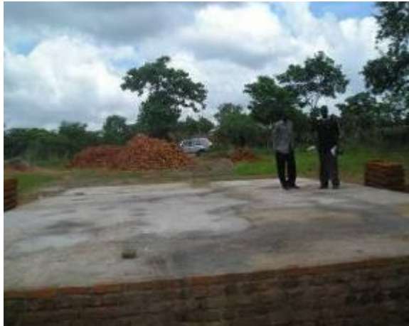
Construction of warehouse at Mkanda
