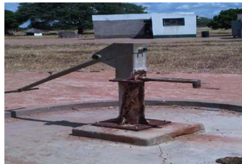
Figure 4: Dried up lake that served for cattle watering and Water pump rusted from salty water
